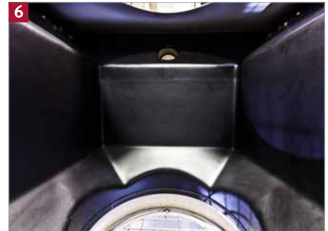
Hopper inside view
